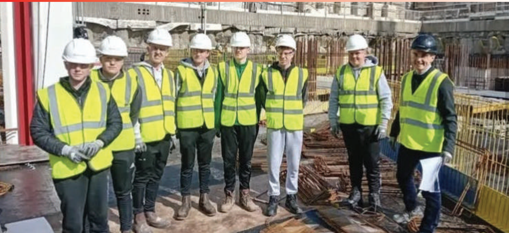
8 students from the 5th Year Leaving Certificate Construction Studies class attended a site visit for Bennett Construction in Kevin Street, Dublin in September.
