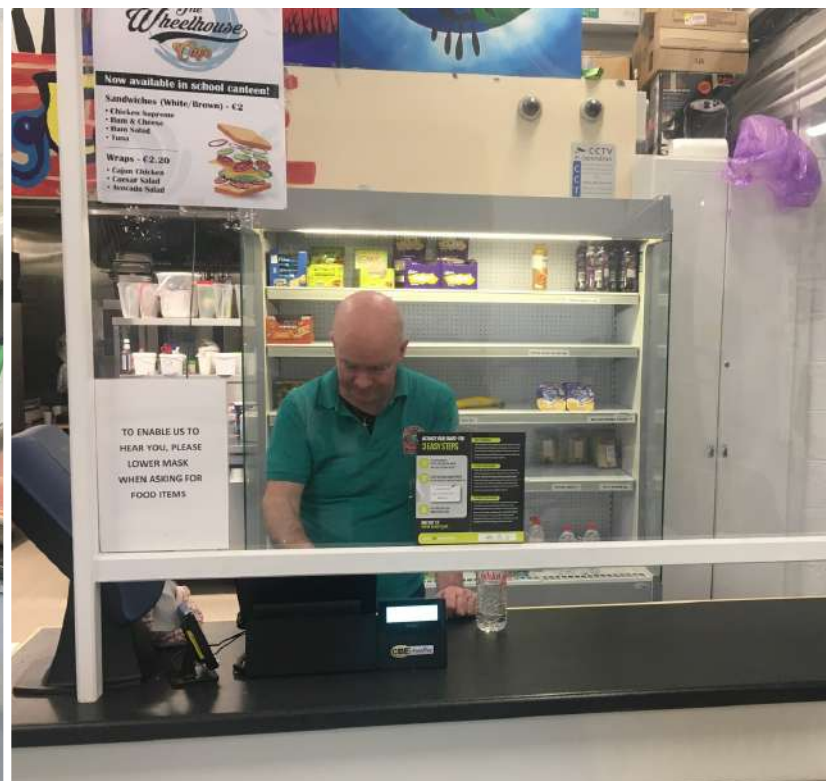
Perspex screens installed at the school canteen for the safety of students and staff.
